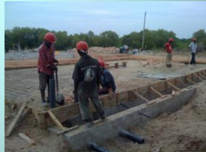
Construction at Dar es Salaam landing station- March 2009
