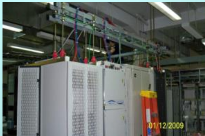
Djibouti Terminal Equipment Being Installed 12 Jan 2009
