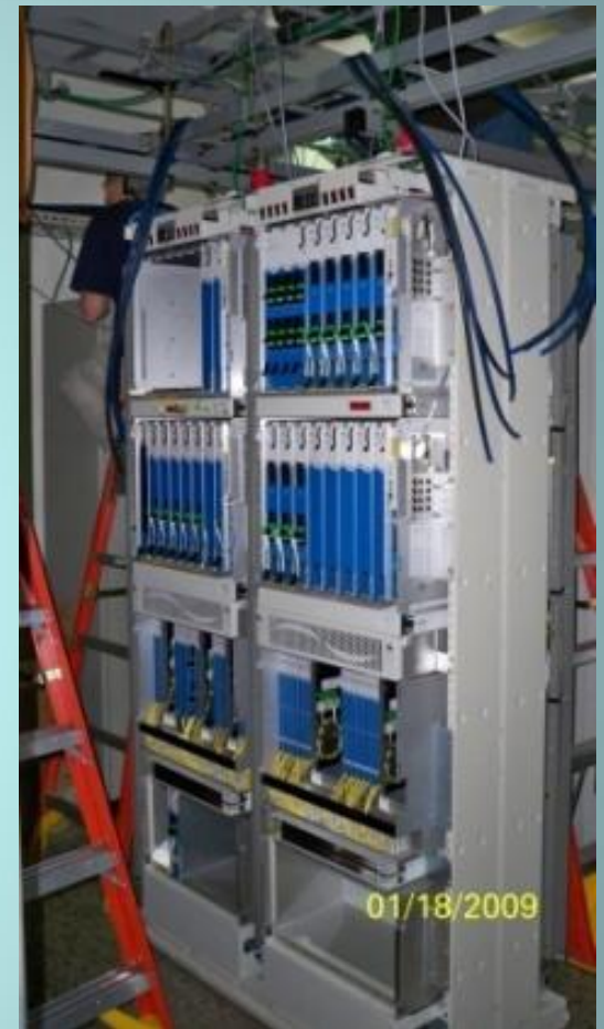
Mumbai Terminal Equipment Being Installed 18 Jan 2009
