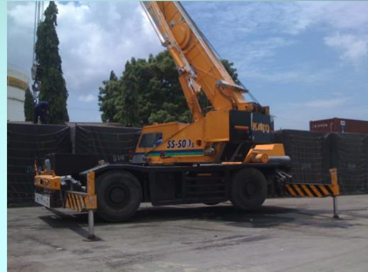
Crane in Tanzania getting ready to move modules- March 2009
