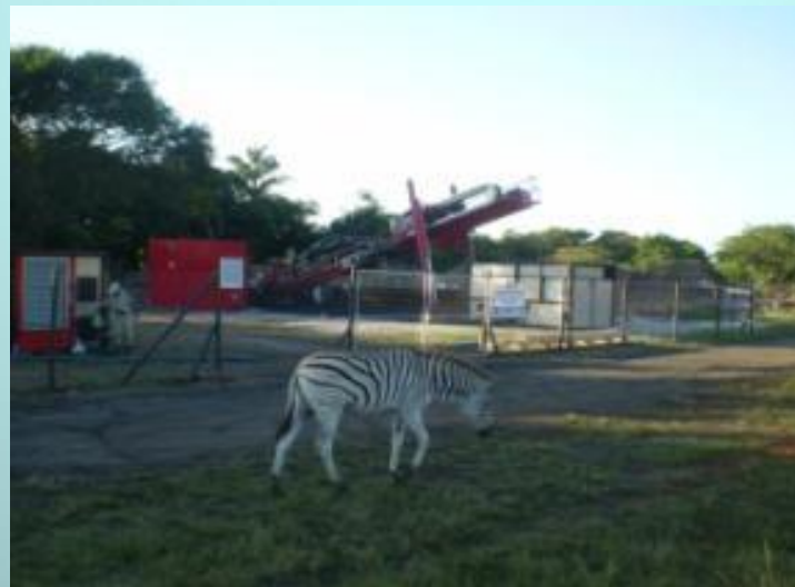
Horizontal Drilling at the Mtunzini landing station- February 2009
